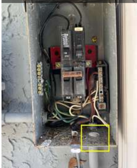
LOCATION: POOL PANEL
