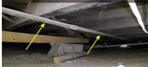
Location: CRAWL SPACE
