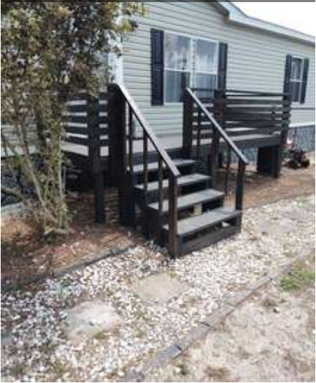
LOCATION: GROUNDS & EXTERIOR
