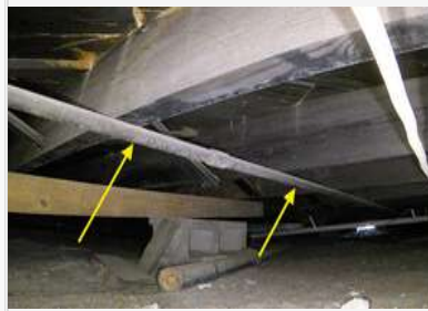
Location: Crawl space
