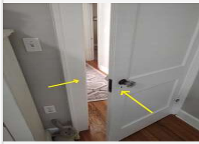
Location: Front bedroom
